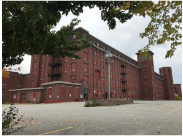
Figure 16 – One of the many former mills in Lewiston-Auburn slated for redevelopment.
